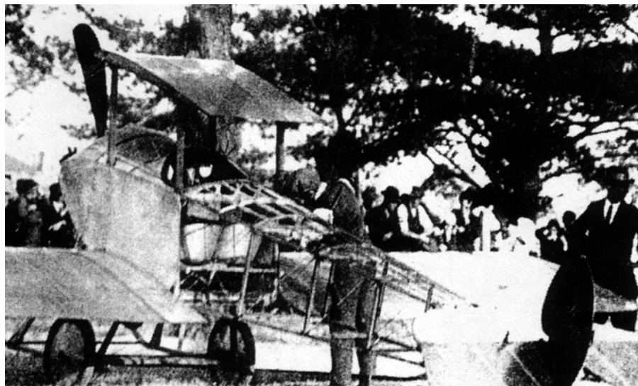
Figure 27 Preparing the plane for the flight. Note that the upper wing of the bi-plane is not yet installed 232
