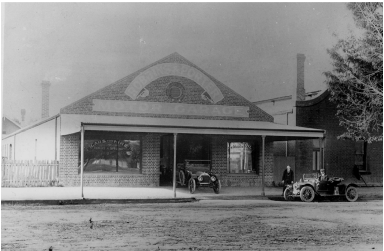
Figure 3 A.D.Robbins' and A.W. Porter's Motor Garage at 532 Kiewa Street photographed in 1913. 35
