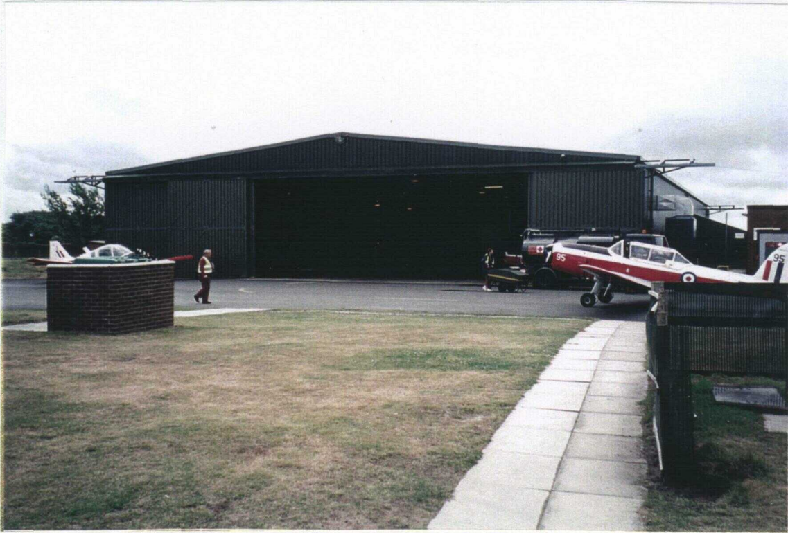
Photo 3.1 External View of Bellman Hangar
