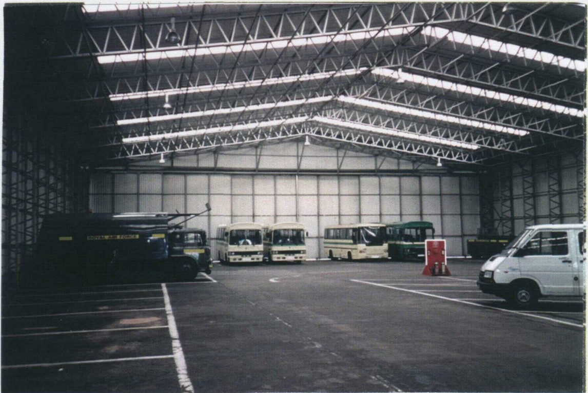
Photo 3.4 Lattice Portal Frame of Type T2 Hangar
