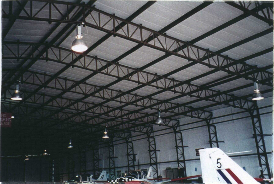
Photo 3.3 Lattice Portal Frame of Bellman Hangar
