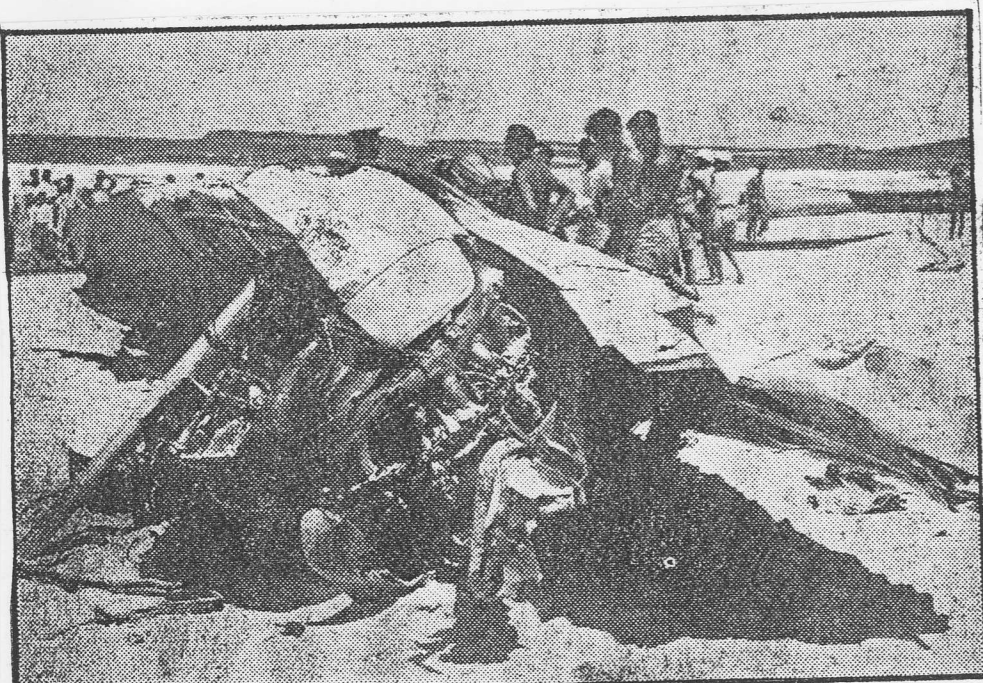
PORTION of the R.A.A.F. plane's wing, covering the engine, was torn from the fuselage in the crash.
