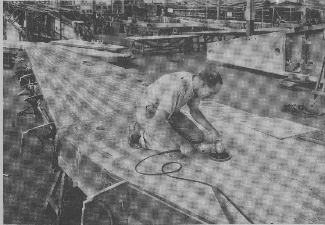
Above: Gouging out wing tank filler hole
