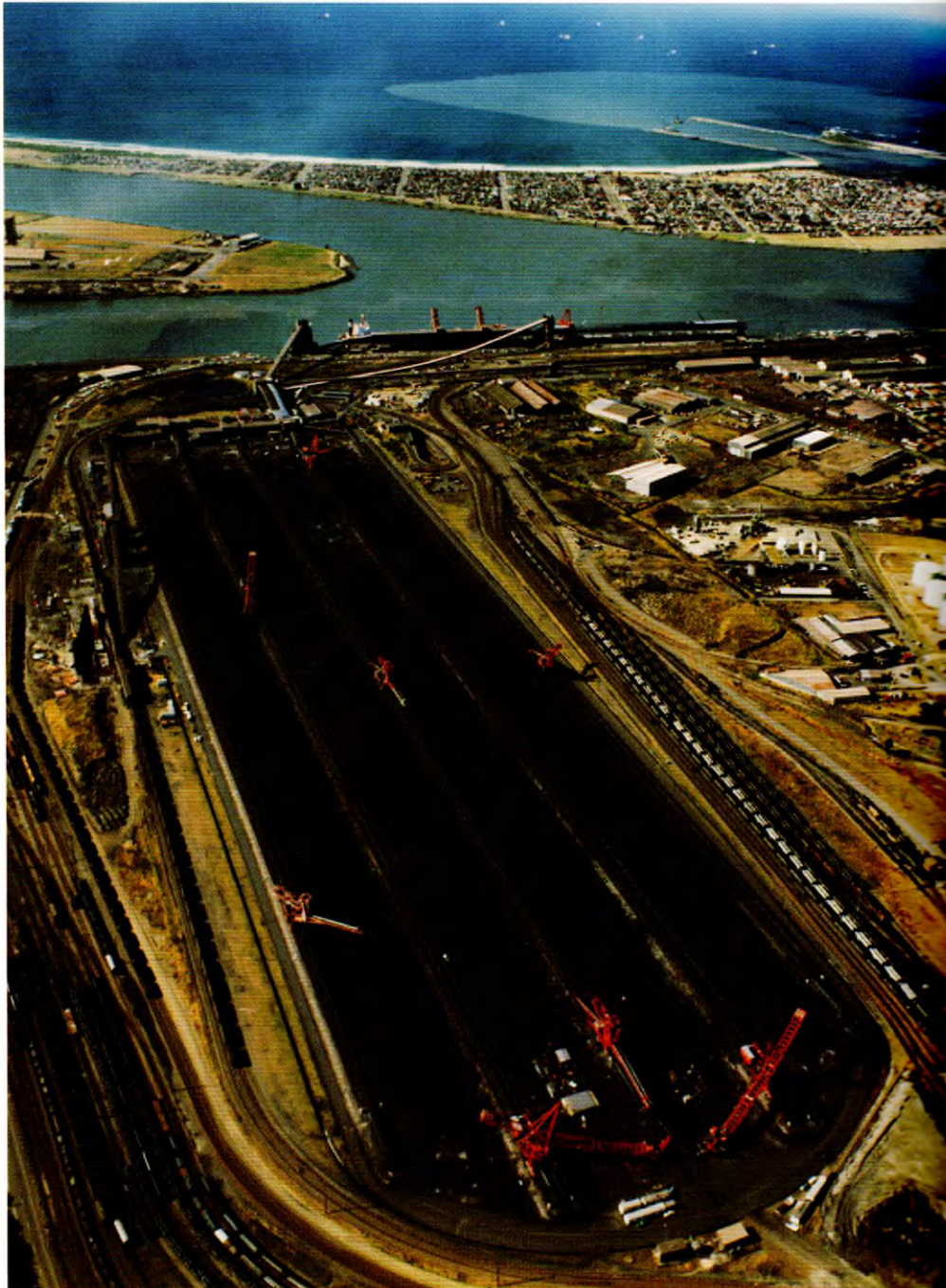
1976. Aerial view of the coal handling and ship loading facility at Port Waratah, Newcastle, NSW, built for the Port Waratah Coal Services (P.W.C.S.).
