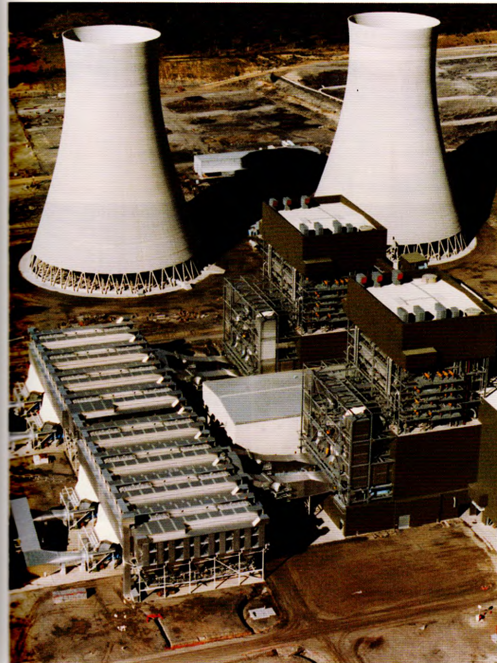
1986. Mount Piper Power Station, NSW. The twin 660MW development contract required the fabrication and erection of 14,000 tonnes of structural steel, along with the assembly of pressure parts, ducting, fuel mills, air heaters, concrete and civil works. The client was
