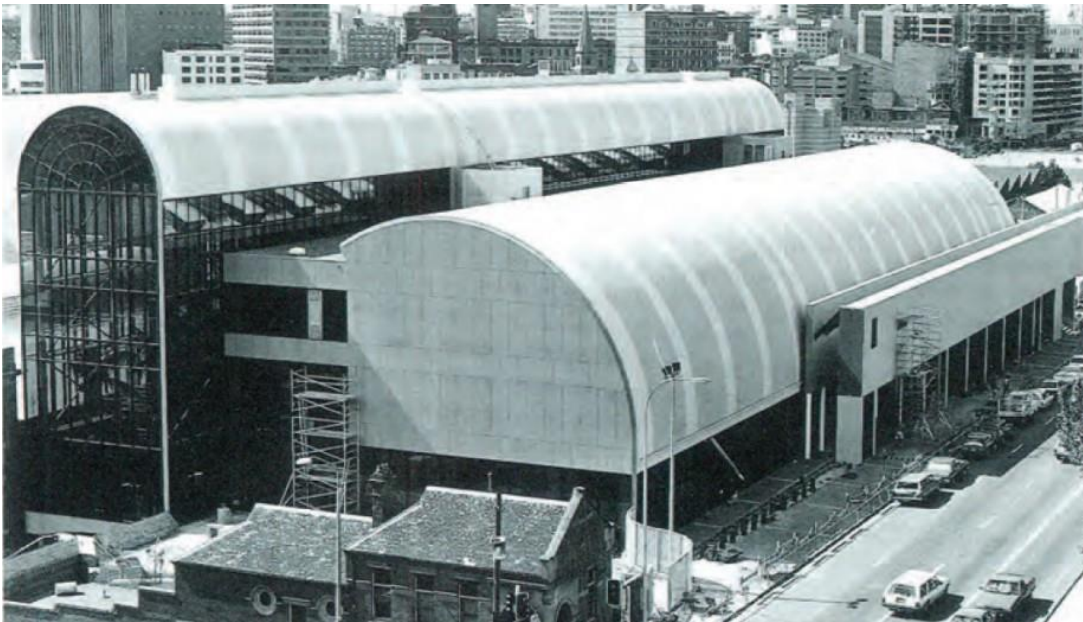
The new building under construction; Ultimo Post Office is in the foreground.
