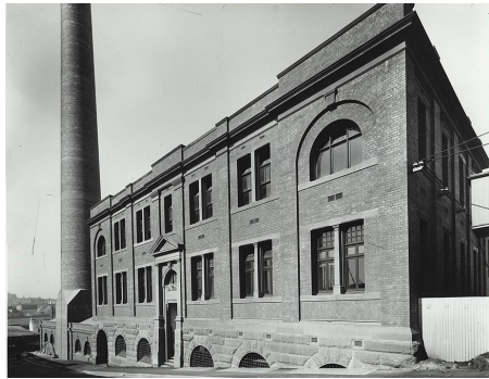
The 1899 Powerhouse. The chimney alone had a million bricks.
