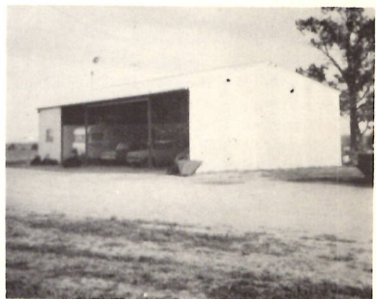
STEEL SHED BY COLEAMBALLY METAL ENGINEERING
