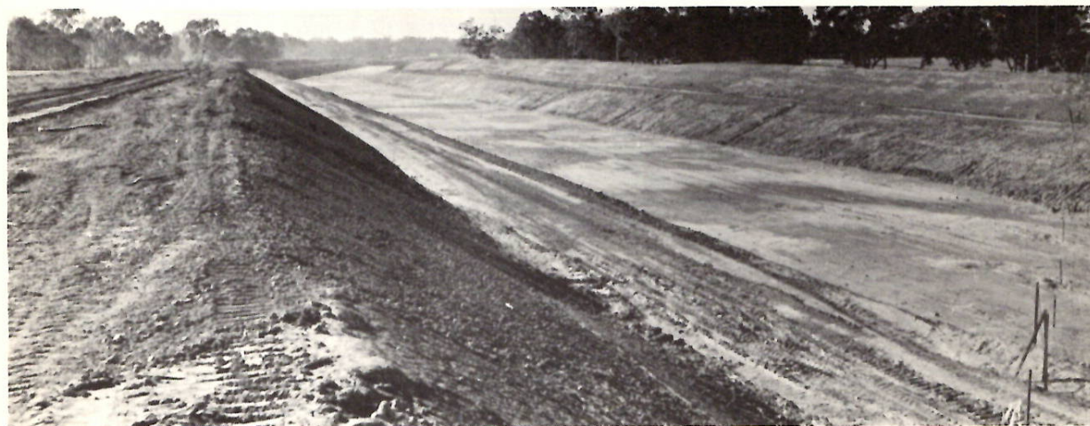
Completed Section of Coleambally Canal – July, 1958. Photo W.C.&I.C.
