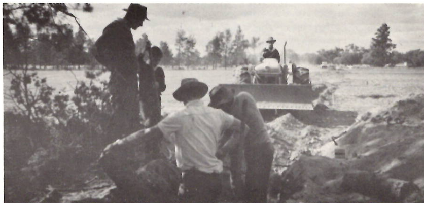
LAYING PIPES ON THE OVAL
